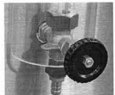
isolation cock (21) and water gauge emptying cock
