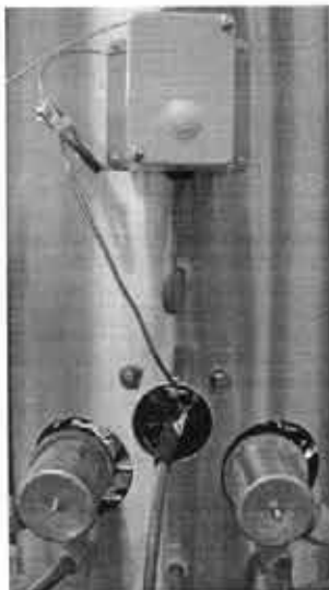
2 heating elements (14), micro heating element and water shortage protection sensor and reset switch (15)
